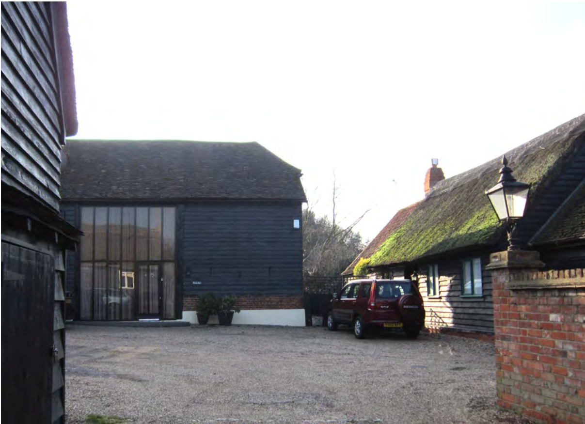
Picture 1.32 Priory Barn, view towards the curtilage from the north
