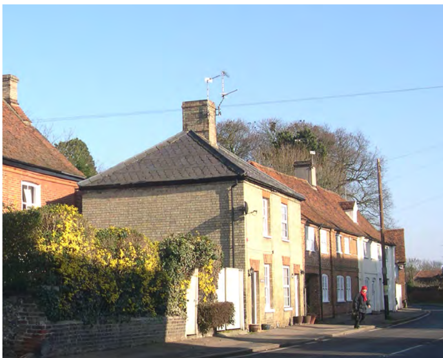
Picture 1.13 Clarob Cottage and Laburnum Cottage, view from the south-west
