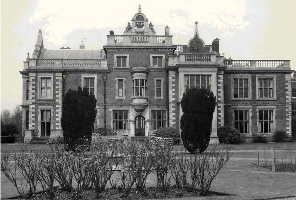
Picture 1.22 Barrington Hall, the front elevation, after 1863
