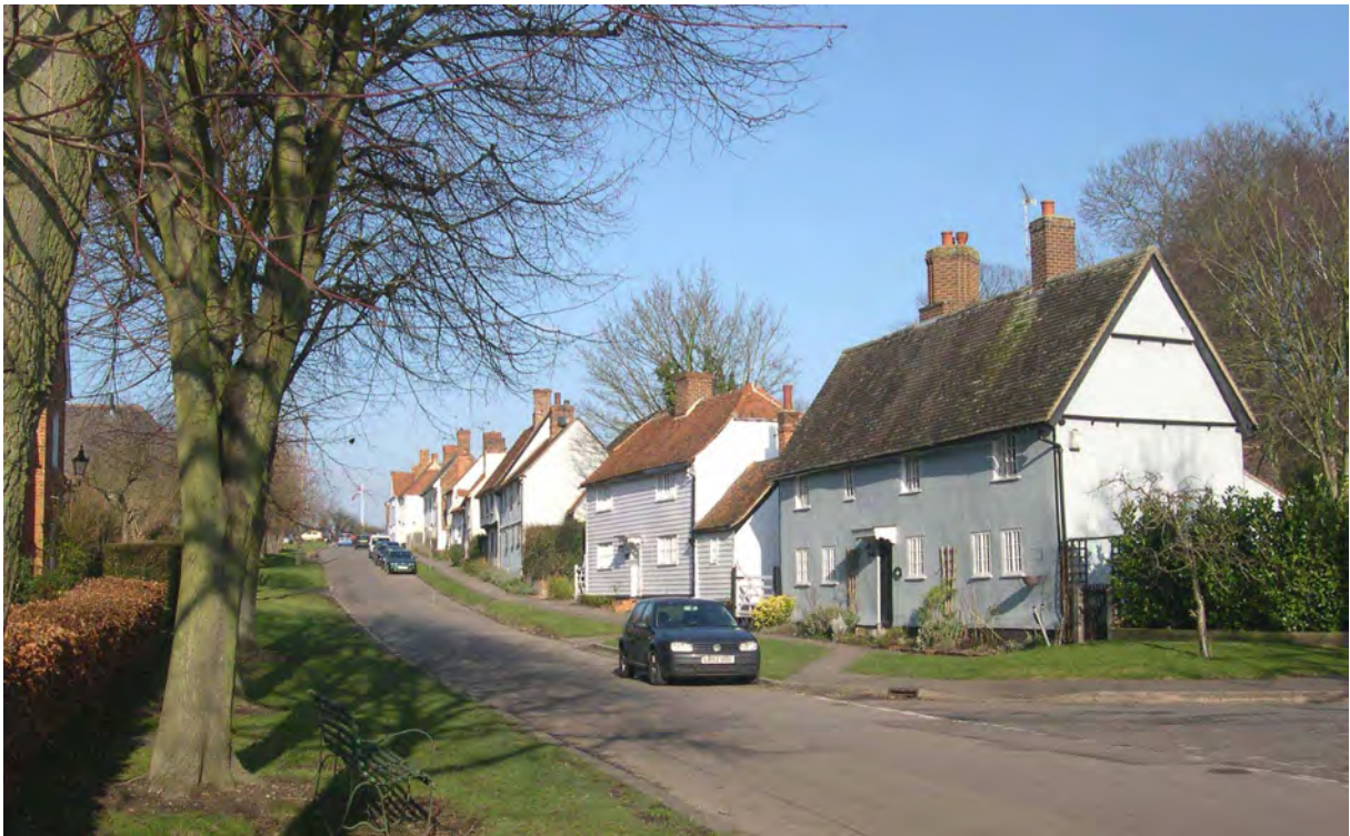
Picture 1.36 Cage End, cottages situated at the southern end of Conservation Area; view to the east
