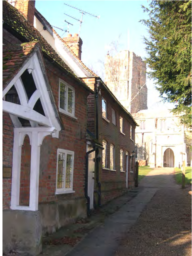
Picture 1.8 High Street; view towards Church Cottage and the footpath leading to the church
